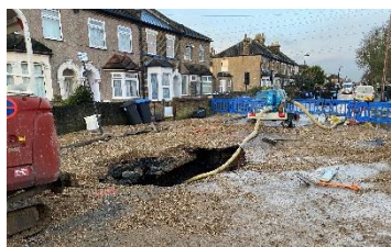
The burst water main created a huge hole and much inconvenience.
